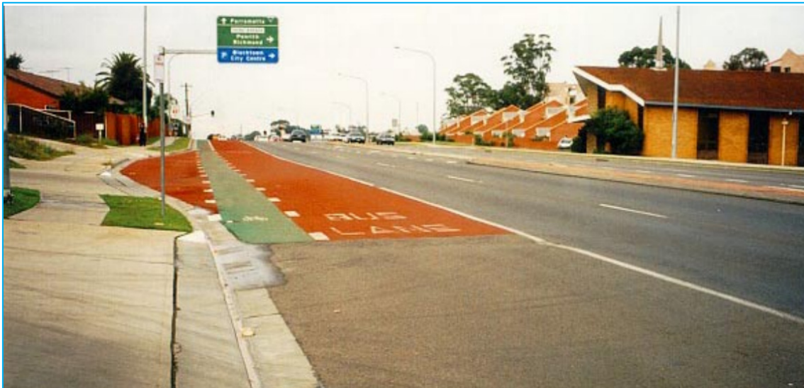
Figure 6.10: On-road Bike Lane. Sunnyholt Road, Blacktown
